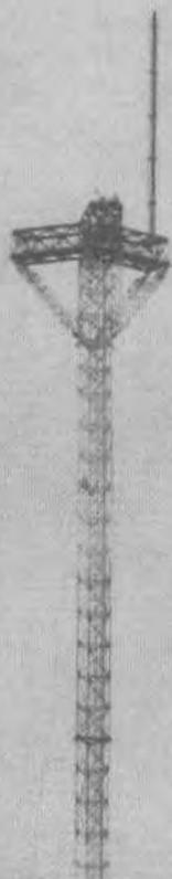
*HC Jefferies Tower crew attaches the base plates for two new antennas in January 2002. Attaching the base plates and antennas was accomplished in 3.5 hours.*
